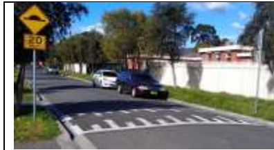
Figure 5: Raised safety platform
