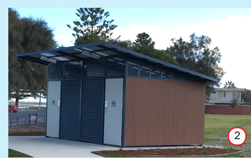
Accessible toilet facilities.
